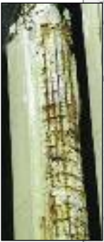
Deterioration of concrete due to improperly designed rebar splices and lack of reinforcement, often leads to premature splice failure.
